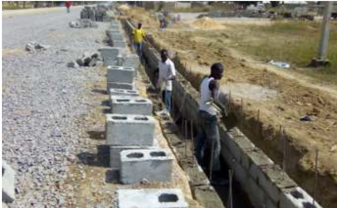
CONSTRUCTION RHS LINE DRAIN AND CARRIAGEWAY SCARIFICATION
