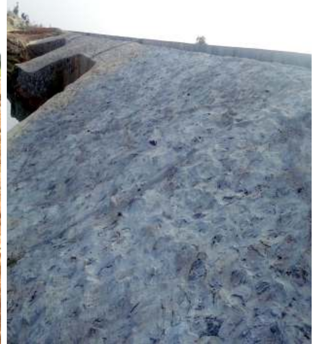
THE ROAD SURFACE AND EMBANKMENT AFTER THE MAINTENANCE WORKS
