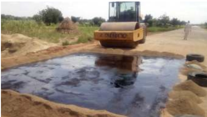
SURFACE DRESSING WORK AT GADAMA CULVERT 1 ST SECTION
