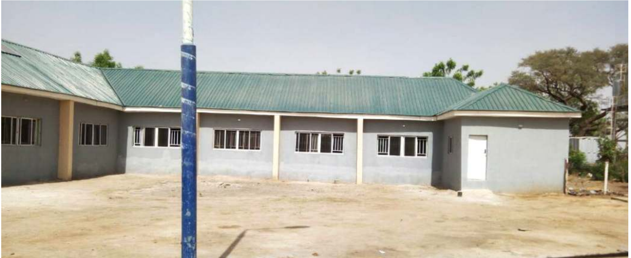
Newly constructed 40 Bed Ward Babura General Hospital
