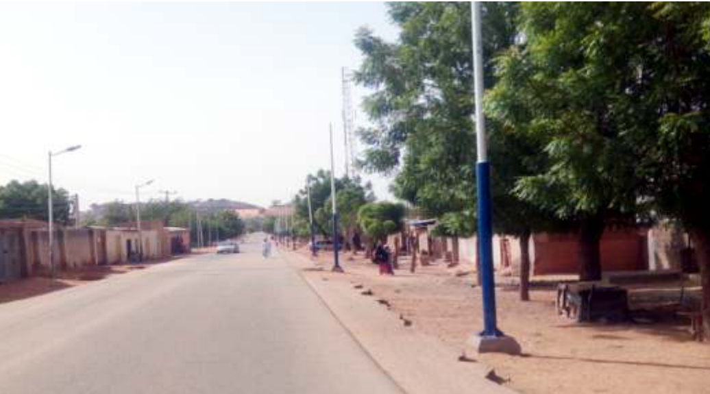
NEWLY INSTALLED INTEGRATED SOLAR STREETLIGHT ALONG GARU (YADI) DUTSE
