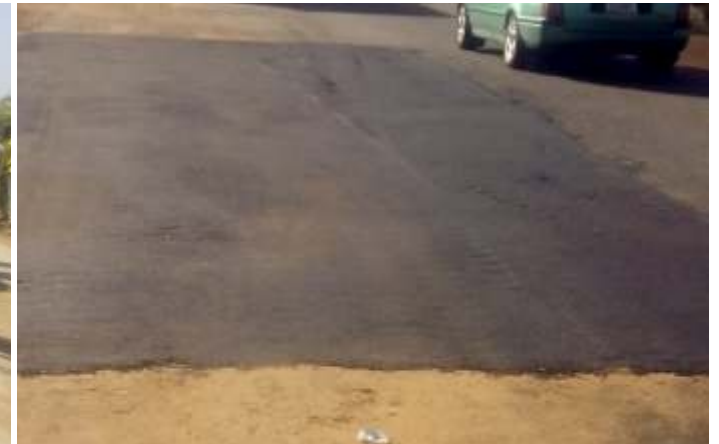
COMPLETED SECTION OF GWARAM- BASIRKA ROAD AFTER THE INTERVENTION WORK
