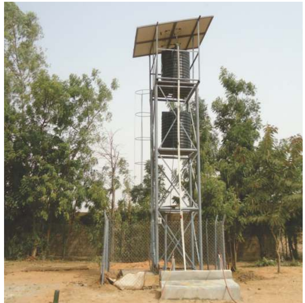
Solar borehole at Great Green Wall project site, Bajoda, Sule Tankarkar LGA
