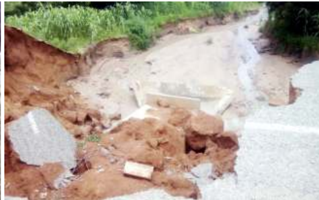
FAILED CULVERT AT GADAMA (NO.2) ON GWARAM - FAGAM ROAD
