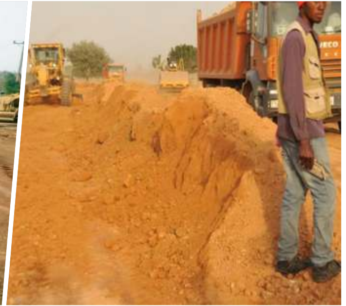
CON'T SPREADING OF SUBBASE MATERIAL
