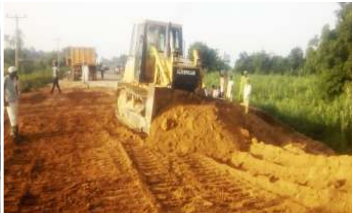
EARTH WORKS IN PROGRESS AT GADAMA CULVERT
