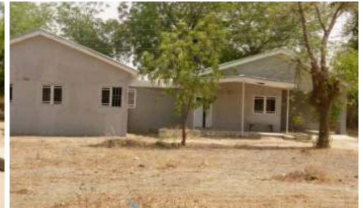
Babura GH Renovated Staff Quarters
