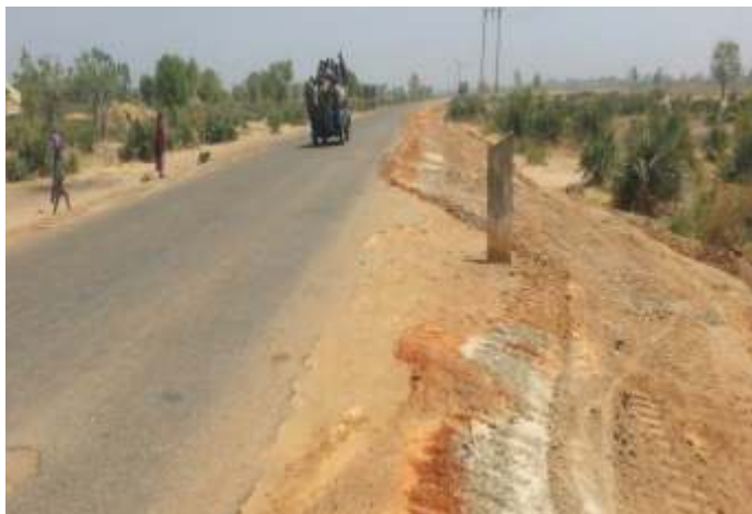
SCARIFICATION OF SHOULDER AND DUMPING OF BASE MATERIAL
