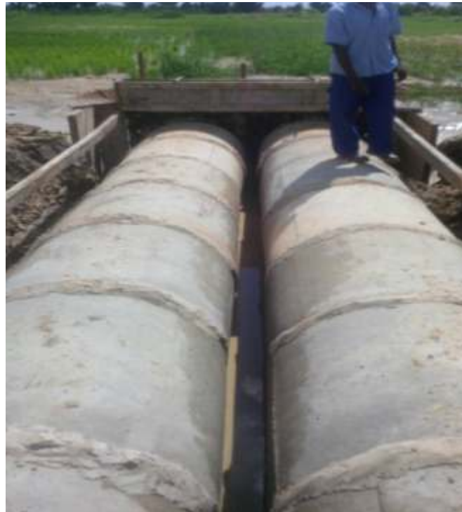
EXCAVATION AND CONSTRUCTION OF 2 CELL RING CULVERT
