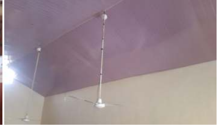
Interior of newly renovated Gwiwa PHC
