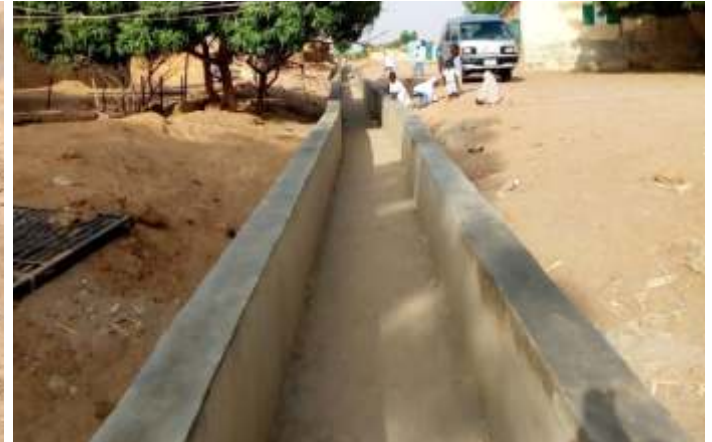
CONSTRUCTION OF DRAINAGES AND CULVERTS AT SAGU TOWN, BUJI LOCAL GOVERNMENT AREA
