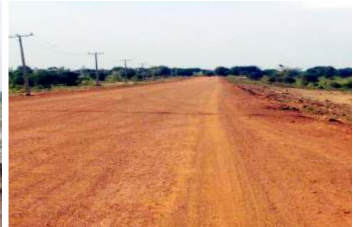
BASE COURSE APPLICATION
