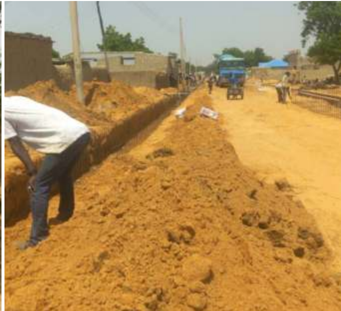
FILLING AND DRAINAGE EXCAVATION IN PROGRESS
