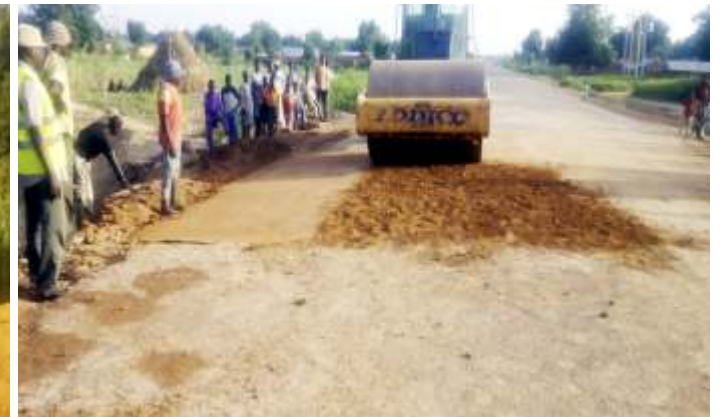
COMPACTION WORK AT GADAMA CULVERT 1 ST SECTION
