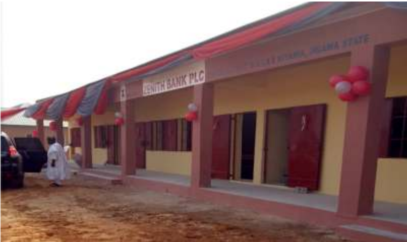
CSR Projects -Commissioning of Zenith Bank project at Kiyawa
