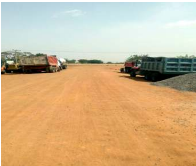
CONSTRUCTION OF KWANAR IDANDUNA – KADOWAWA - 22.4KM
