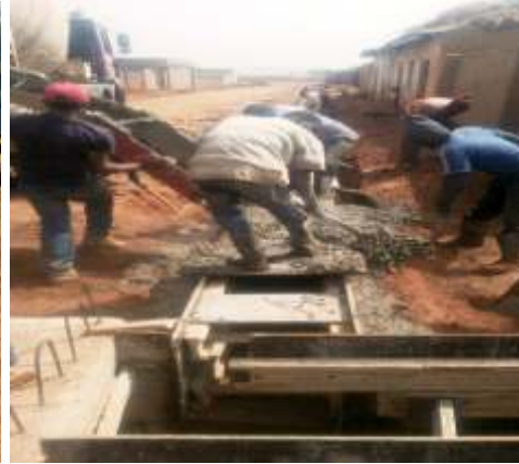
CONCRETE DRAINAGE WORKS
