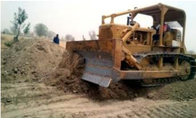
DUMPING AND SPREADING OF FILL MATERIAL
