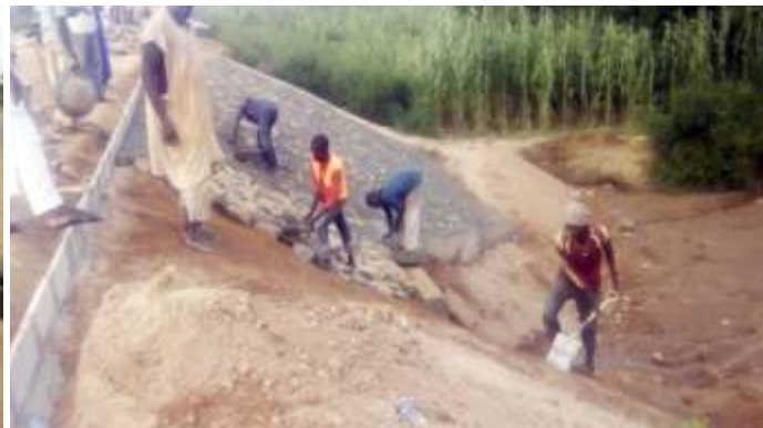
STONE PITCHING WORK AT GADAMA CULVERT
