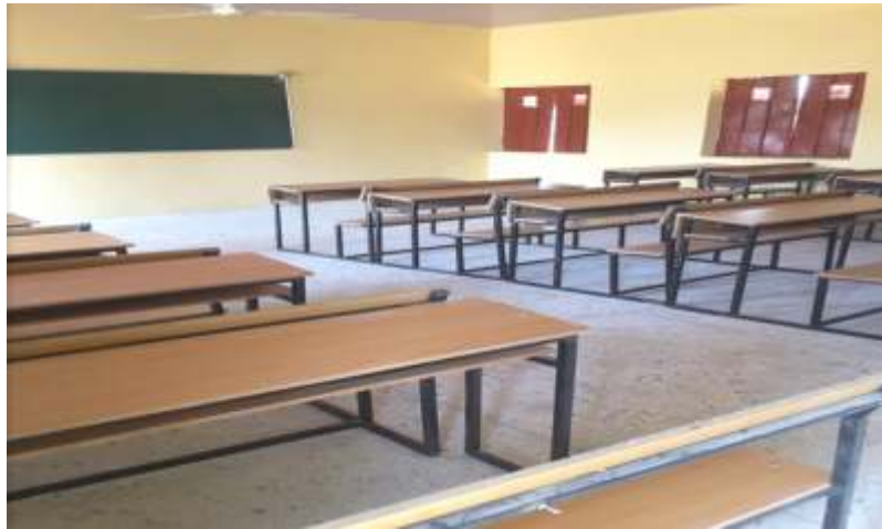
Classroom at Kiyawa constructed by Zenith Bank
