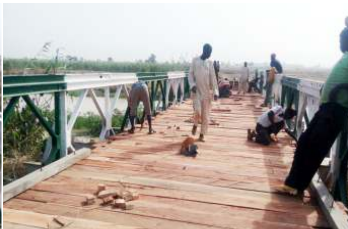
INSTALATION OF NEW TIMBER DECKING
