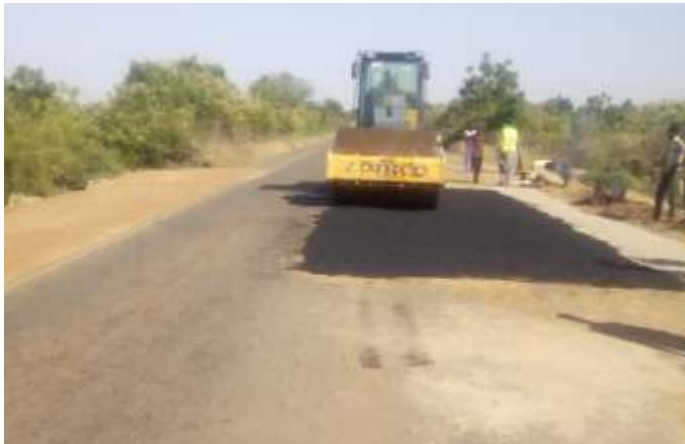
PRIMING AND ASPHALTIC CONCRETE RESEALING OF THE FAILED SECTION ON GWARAM-BASIRKA ROAD
