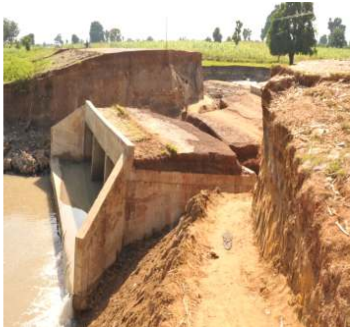
DAMAGED 6 CELL BOX CULVERT
