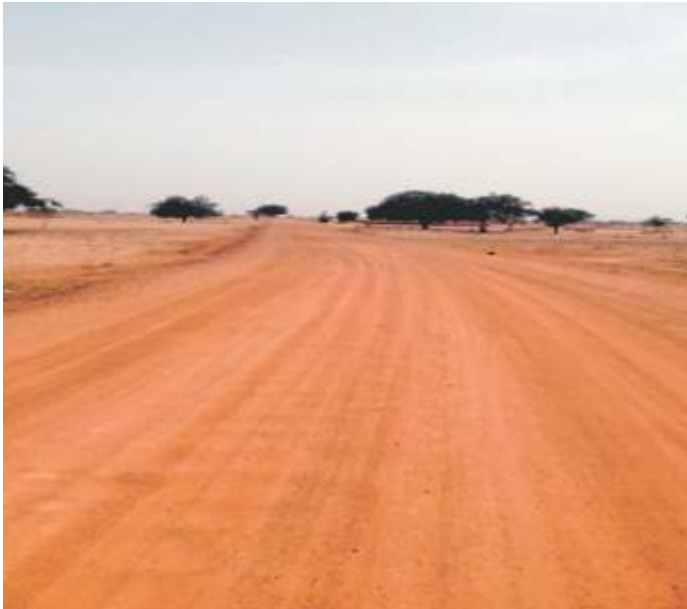
CONSTRUCTION OF LAMBAR ZAUMAR MAHAUTA – DUWIGI – GWIWA ROAD - 15KM
