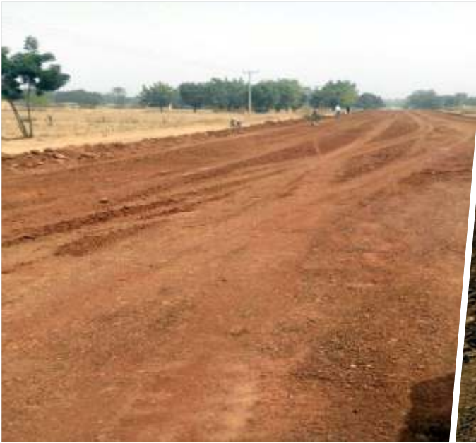
SPREADING OF LATERITE SUBBASE MATERIAL AND DUMPING OF BASE MATERIAL
