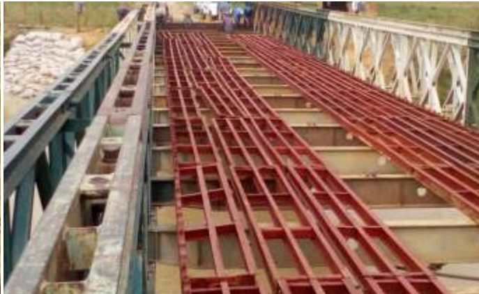
RE ASSEMBLING STRAINERS
