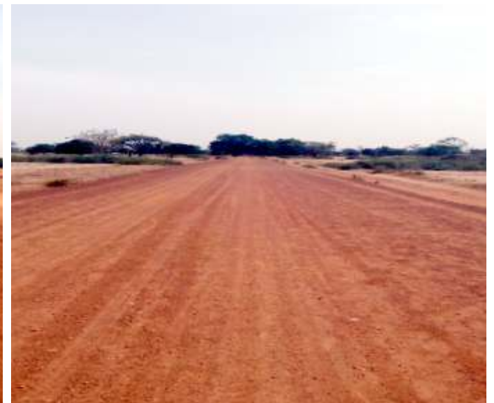
CONSTRUCTION OF TSAMIYA KWANCE – JAMUS – RATAYE - LAMINTANI - 15,1KM
