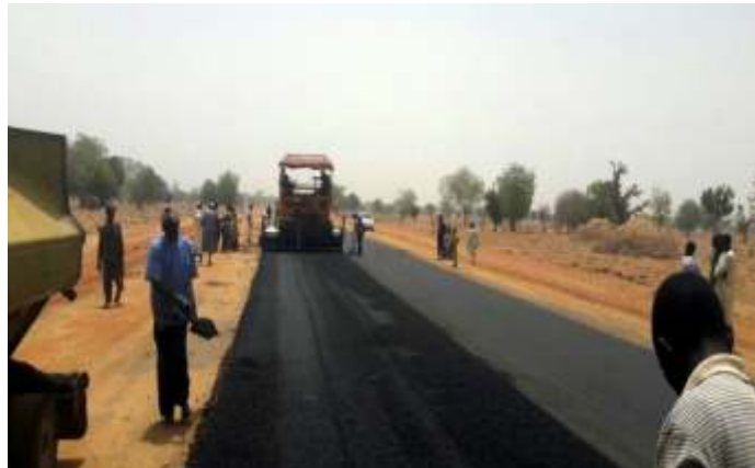
ASPHALT PAVING AND COMPLETED ROAD SECTION
