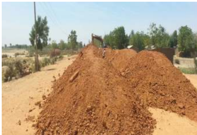
SCARIFICATION OF SHOULDER AND DUMPING OF BASE MATERIAL
