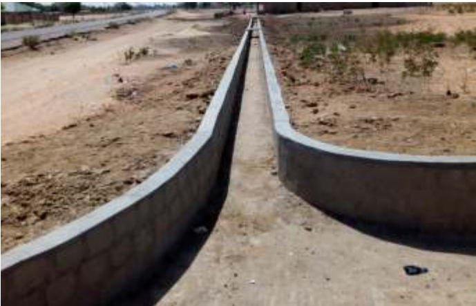
CONSTRUCTION OF DRAINAGES AND CULVERTS AT ASHURAN CHIROMA TOWN, KAFIN HAUSA LOCAL GOVERNMENT AREA
