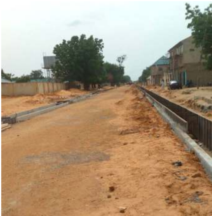
FINISHED DRAINAGE SECTION
