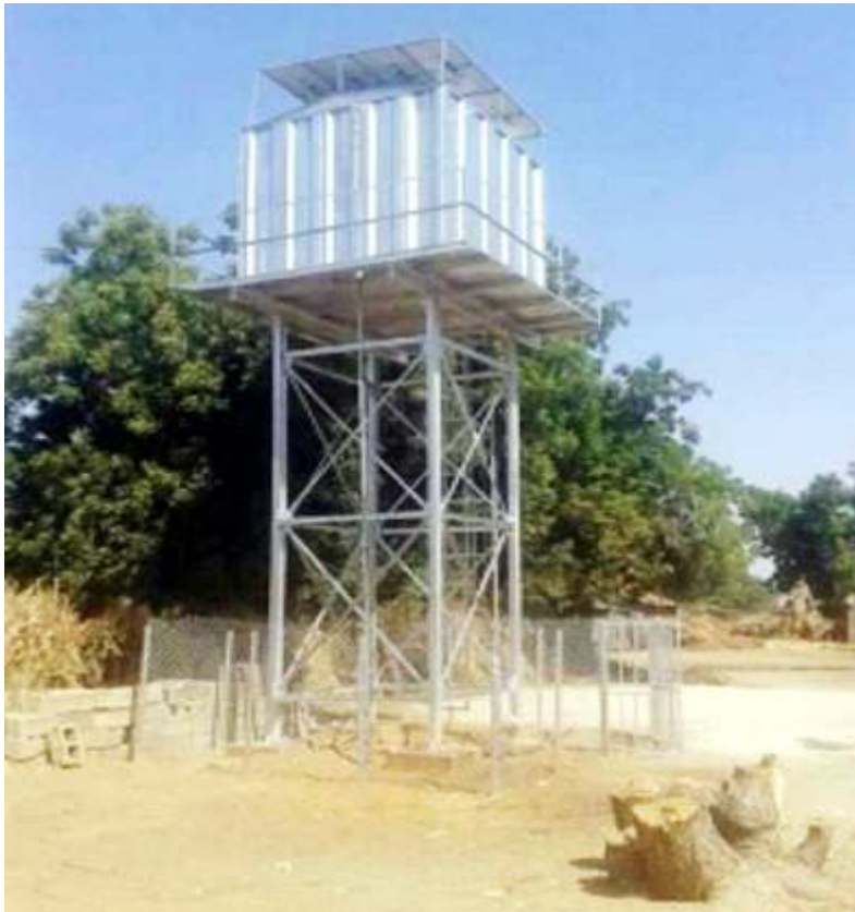
ONE OF THE NEWLY CONSTRUCTED SOLAR POWERED WATER SUPPLY SCHEME AT KWARTA IN RINGIM LGA (MDGS)
