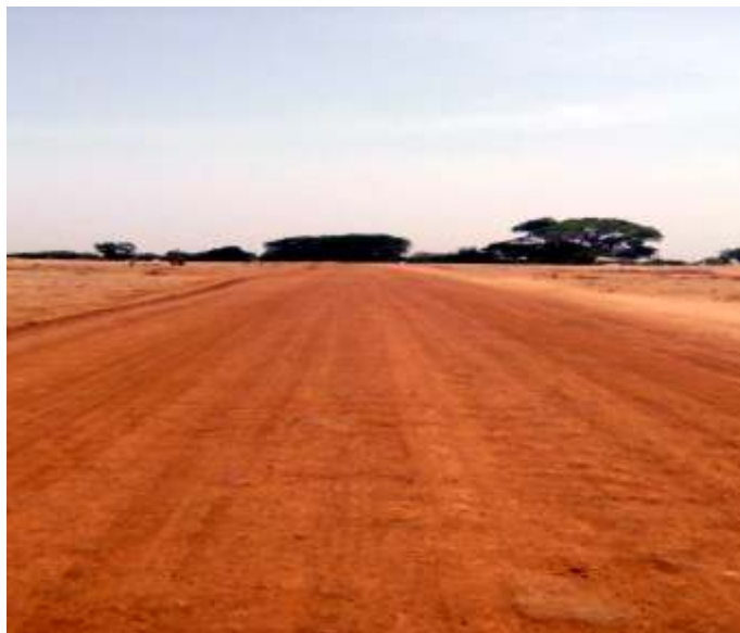
CONSTRUCTION OF MALLAM MADORI- DAKIDO - 5.4KM
