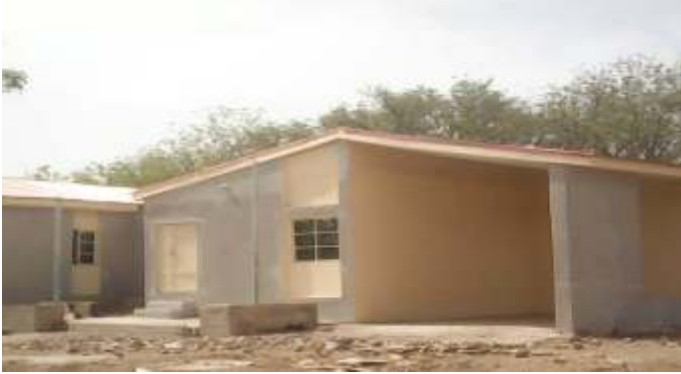
Renovated teachers quarters at GGASS Babura
