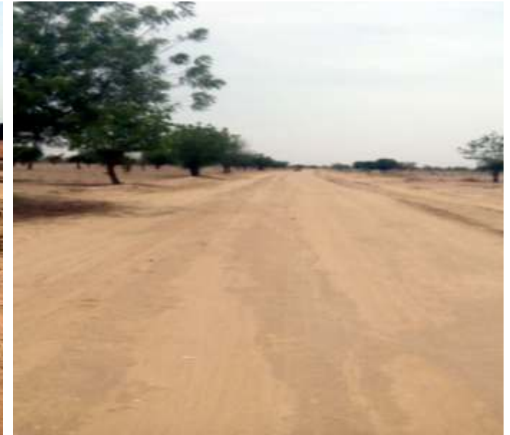
CONSTRUCTION OF GUMEL – GARIN GAMBO ROAD - 7KM
