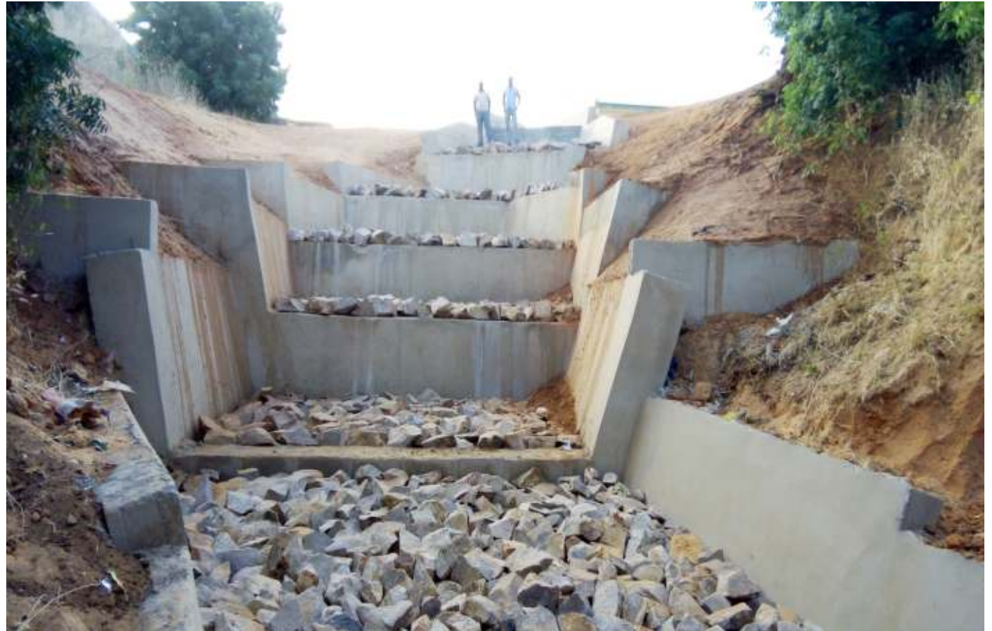
COMPLETED RETAINING WALL
