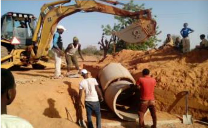
CONSTRUCTION OF CULVERT
