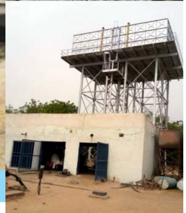
REHABILITATED GENERATOR ROOM AND 200M 3 OVERHEAD TANK AT HADEJIA MAIN PUMP HOUSE
