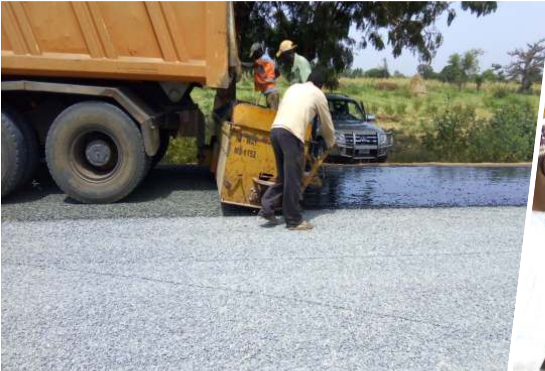
SURFACE DRESSING IN PROGRESS
