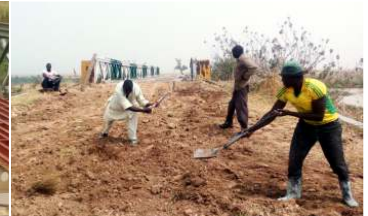
FILLING AND COMPACTION OF APPROACHES
