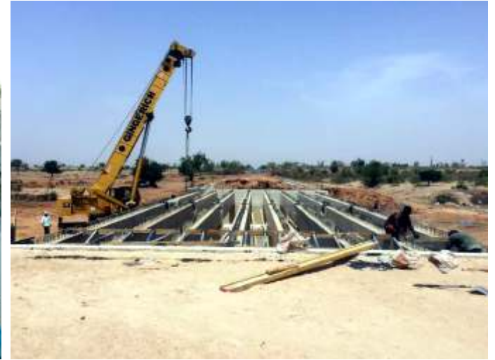
INSTALLATION OF BEAM GIRLDRS
