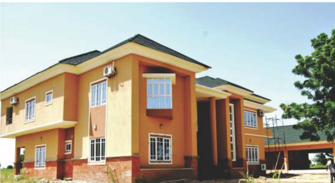
Side view of the completed VC lodge
