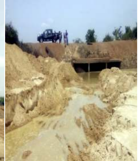
DREDGING OF SAGI CULVERT ON GWARAM-BASIRKA ROAD
