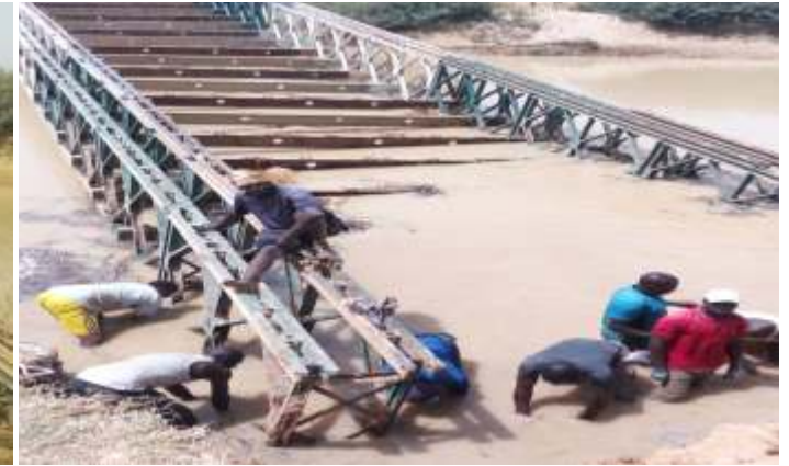
JACKING IN PROGRESS
