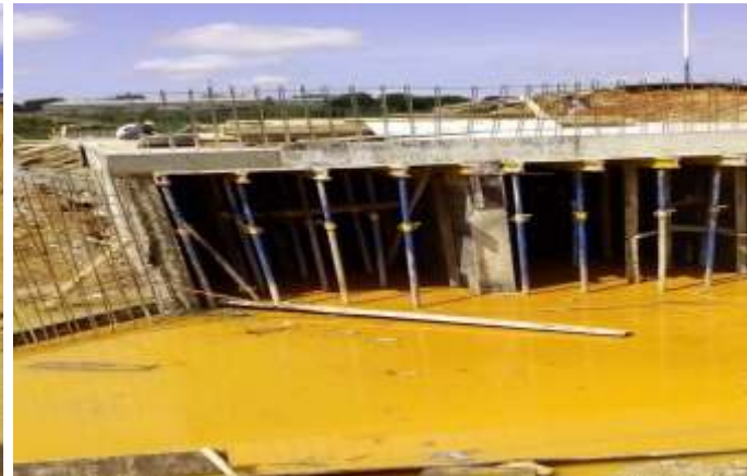
Kazaure Bridge Construction Works in progress
