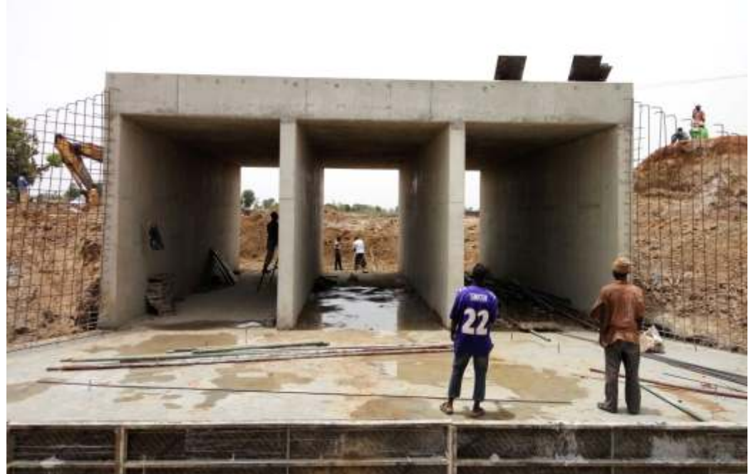
TSAMIYA – YALWANDAMAI- BIRNIN KUDU ROAD WORK IN PROGRESS
