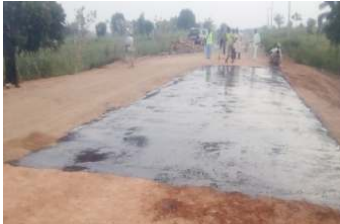
PRIMING AT GADAMA CULVERT
