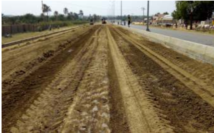
CONSTRUCTION RHS LINE DRAIN AND CARRIAGEWAY SCARIFICATION
