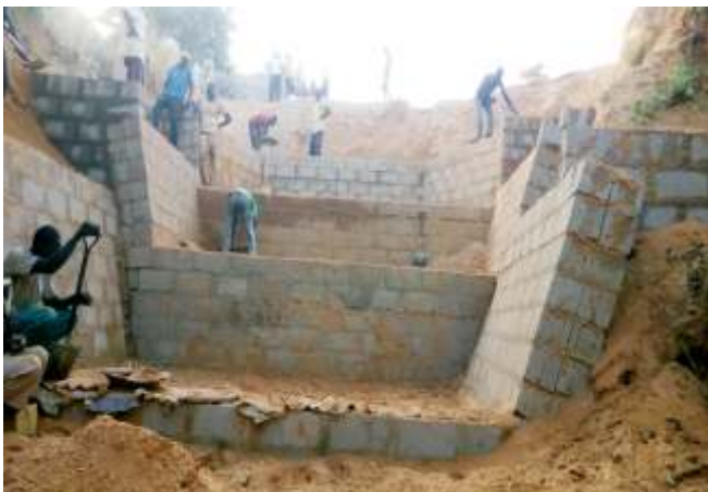
CONSTRUCTION OF RETAINING WALL
