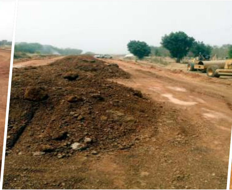
SPREADING OF LATERITE SUBBASE MATERIAL AND DUMPING OF BASE MATERIAL
