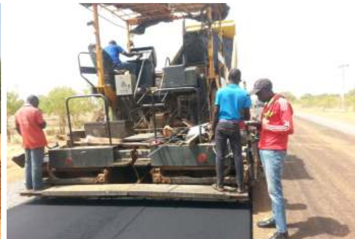
ASPHALT PAVING
