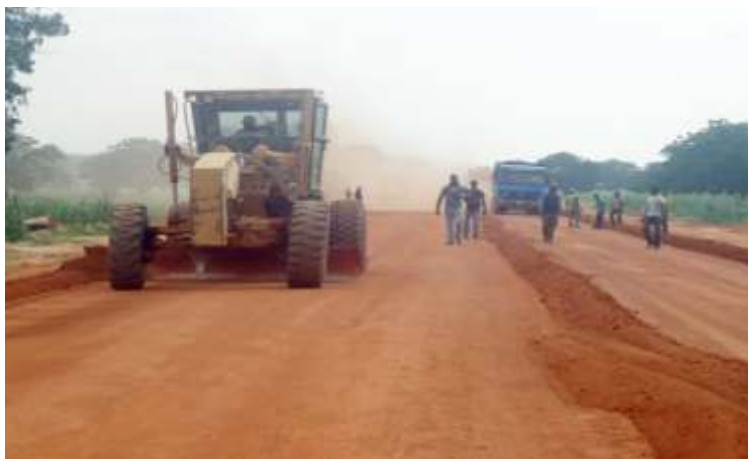
CLEARANCE AND GRADING OF SUBBASE
