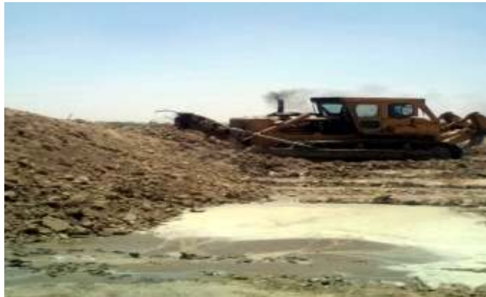
DUMPING AND SPREADING OF FILL MATERIAL
