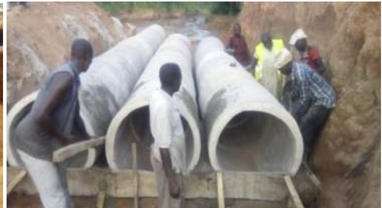
WORKS IN PROGRESS AT GADAMA CULVERT(NO.2)
