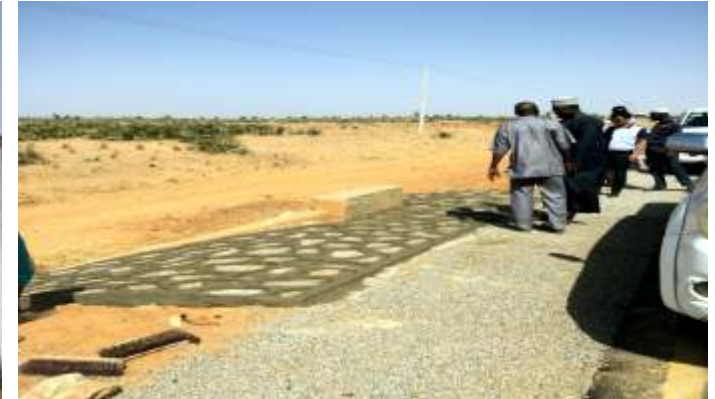
STONE PITCHING (PROTECTION OF EMBANKMENT)
