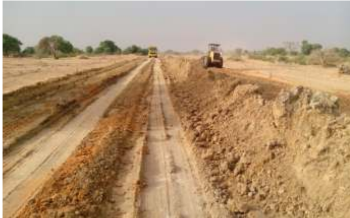
GRADING OF FILLING MATERIAL
