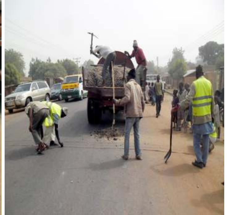
CONSTRUCTION OF SPEED BREAKERS IN COLLABORATION WITH FERMA AND FRSC AT APPROPRIATE LOCATION ON KANO – BIRNIN KUDU – KARI ROAD
