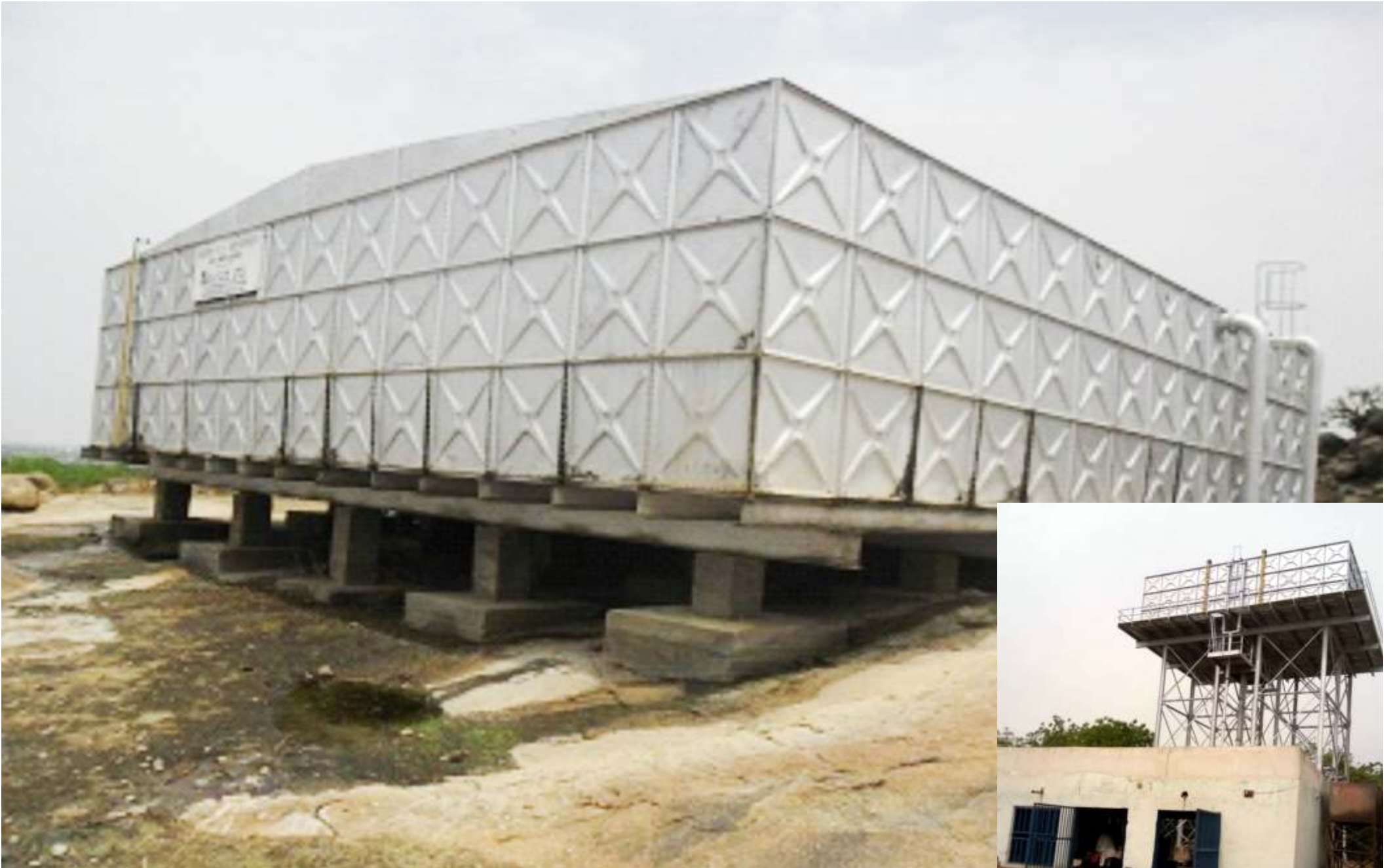
1 MILLION M 3 CAPACITY HILLTOP SURFACE TANK, ALONG KIYAWA ROAD DUTSE AFTER REHABILITATION
