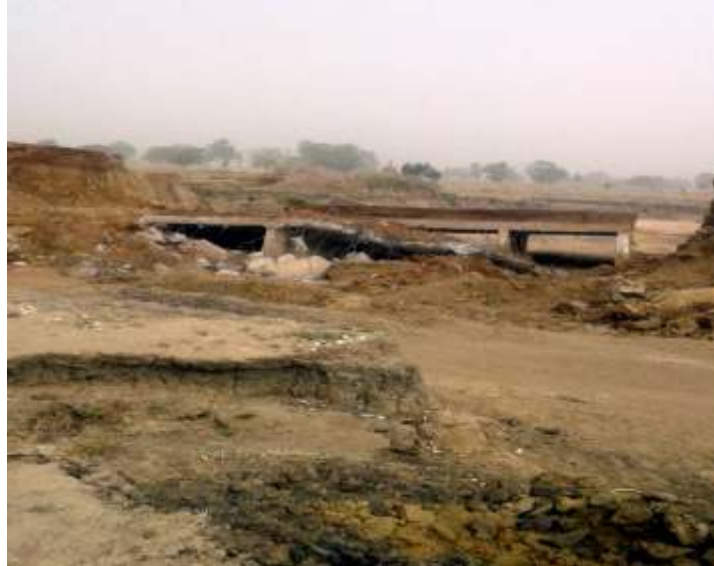
DEMOLITION OF THE FAILED CULVERTS
