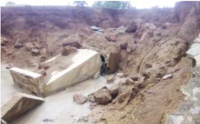
FAILED CULVERT AT GADAMA (NO.2) ON GWARAM - FAGAM ROAD
