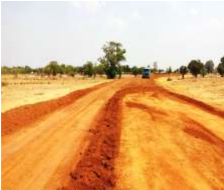
SPREADING OF SUB BASE MATERIAL
