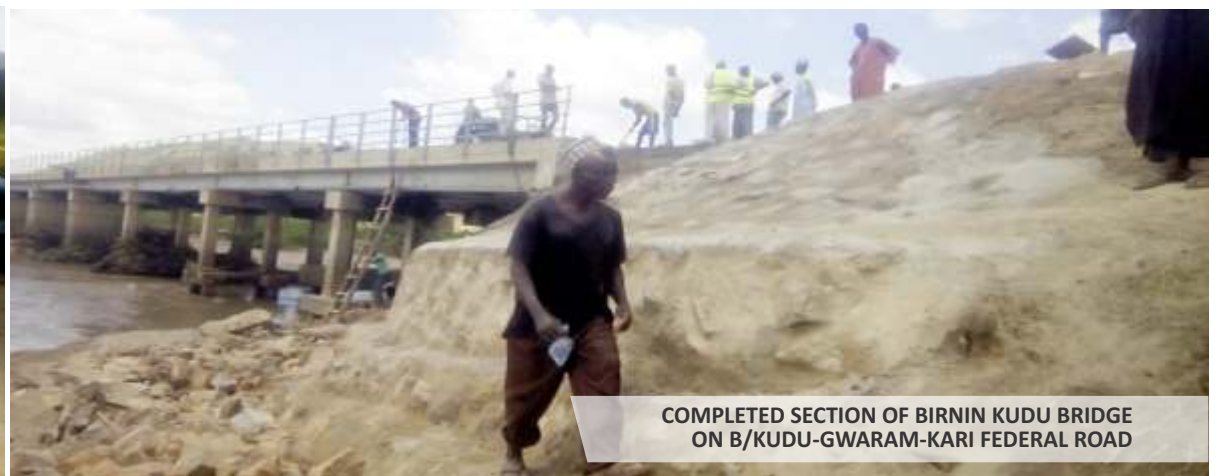
STONE PITCHING WORK AT BIRNIN KUDU BRIDGE
