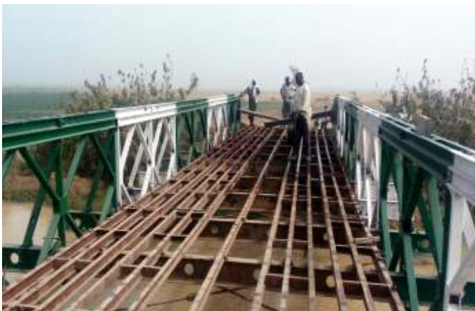
REPAINTING AND REPAIR OF STRAINERS
