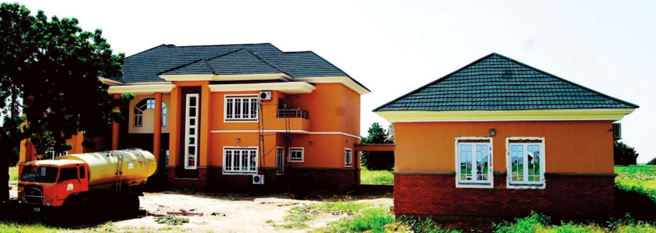
Front view of the completed VC lodge
