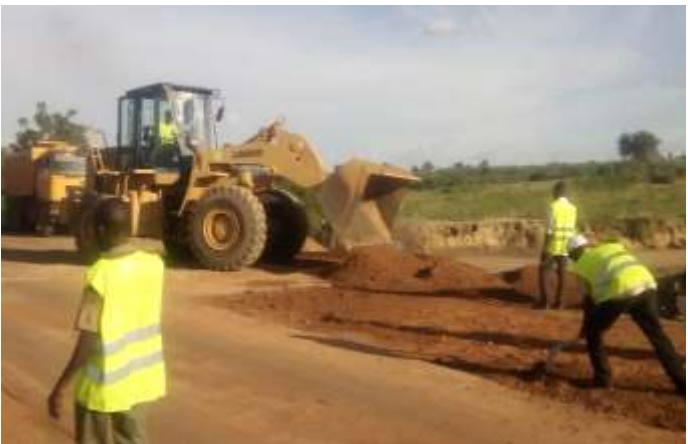
WORKS IN PROGRESS AT GWARAM – BASIRKA ROAD
