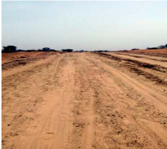
CONSTRUCTION OF SHAFAR – GIDAN SANI – DAGUZAU ROAD - 17.4KM
