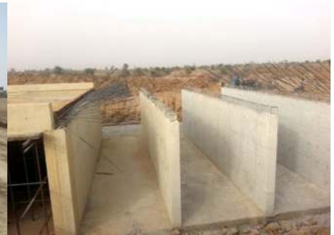
3 CELL BOX CULVERT UNDER CONSTRUCTION
