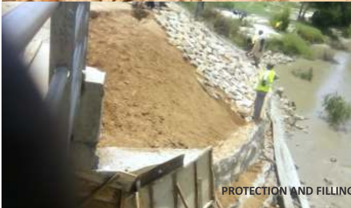
WASHED OUT SECTION OF BIRNIN KUDU BRIDGE
