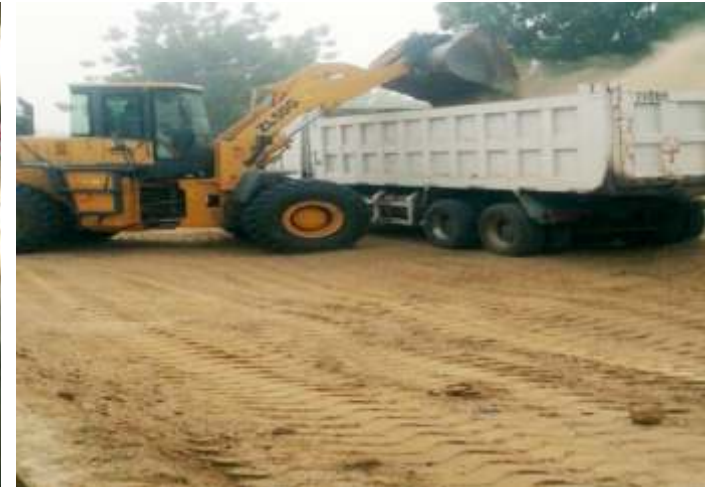
REMOVAL OF UNSUITABLE
