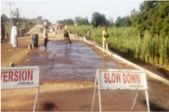
PRIMING AT GADAMA CULVERT
