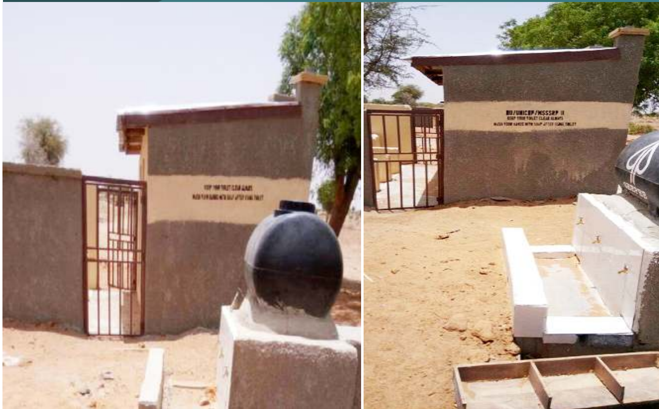
Newly constructed VIP Latrine at Babuwa Primary School M/Madori
