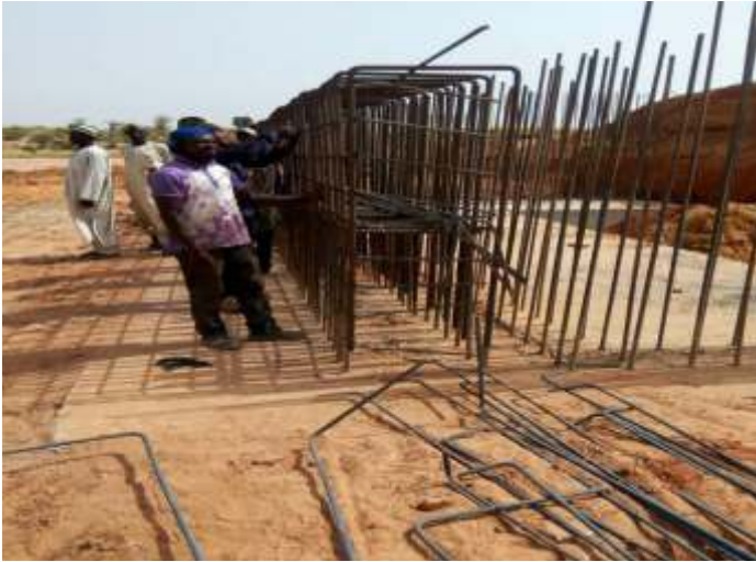
ARRANGEMENT OF REINFORCEMENT FOR ABUTMENT
