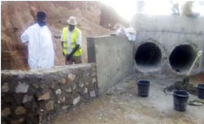
DIRECTOR ENGINEERING JIRMA INSPECTING PROTECTION WORK GADAMA CULVERT
