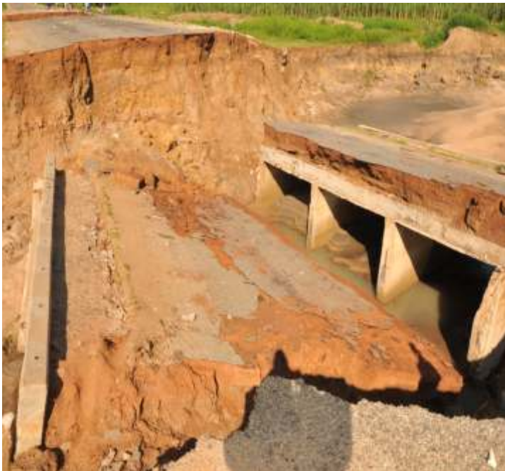
DAMAGED 6 CELL BOX CULVERT
