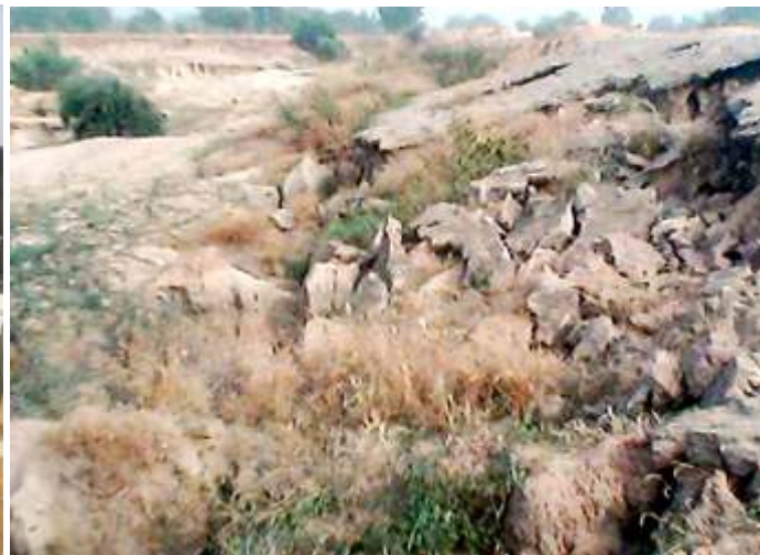
FAILED EMBANKMENT THREATENING THE PAVEMENT AT KADAITA
