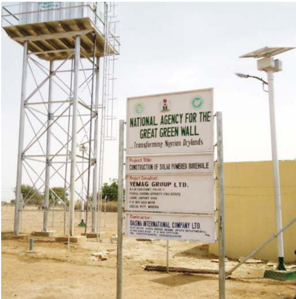
Solar borehole at Great Green Wall project site, Takure, Sule Tankarkar LGA
