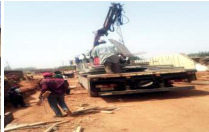
RELOCATION OF UTILITIES
