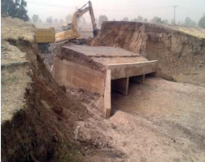
DEMOLITION OF THE FAILED CULVERTS
