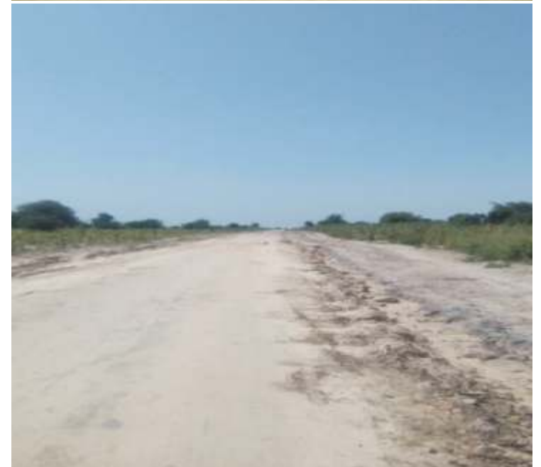
CLEARANCE AND FILLING IN PROGRESS
