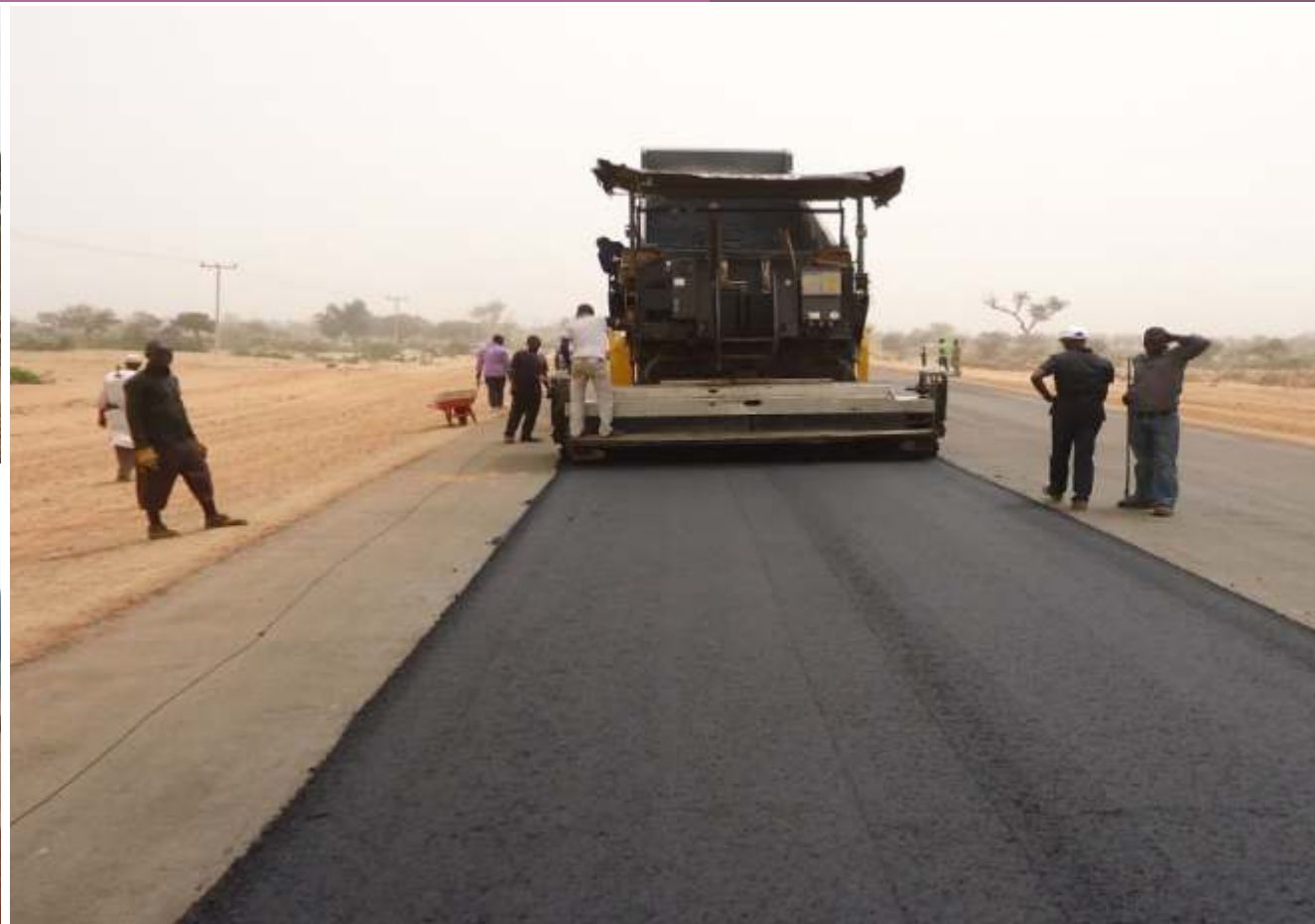
ASPHALTIC PAVING AND FINISHING
