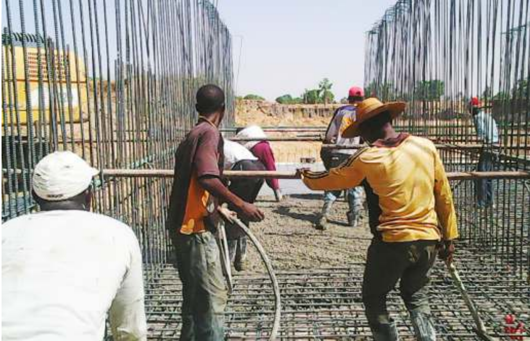
RECONSTRUCTION WORK ON PROGRESS
